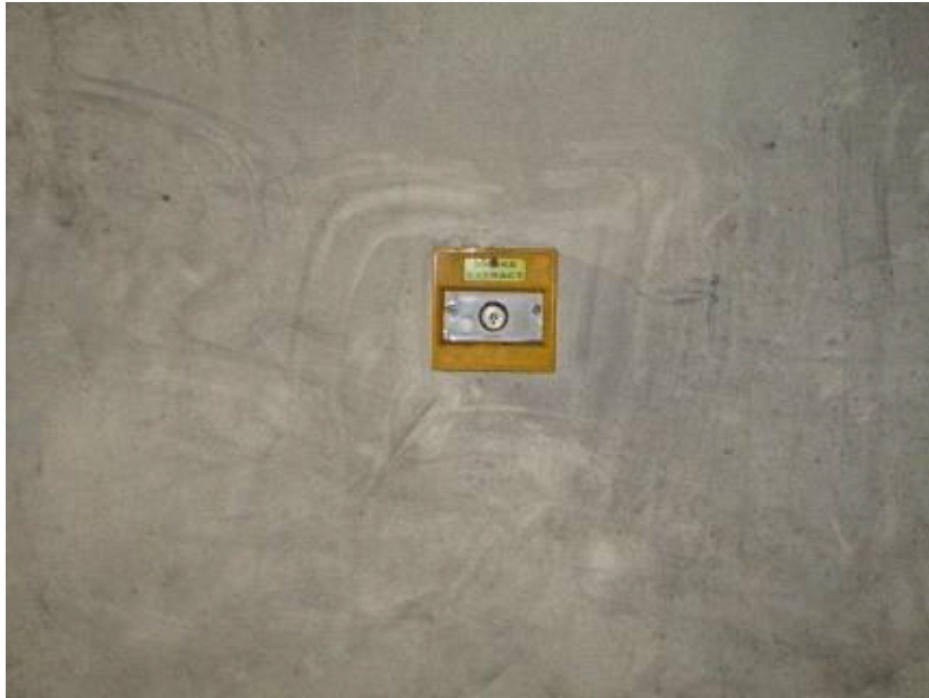
Figure J.16: Smoke ventilation system override switch on Level 4.
