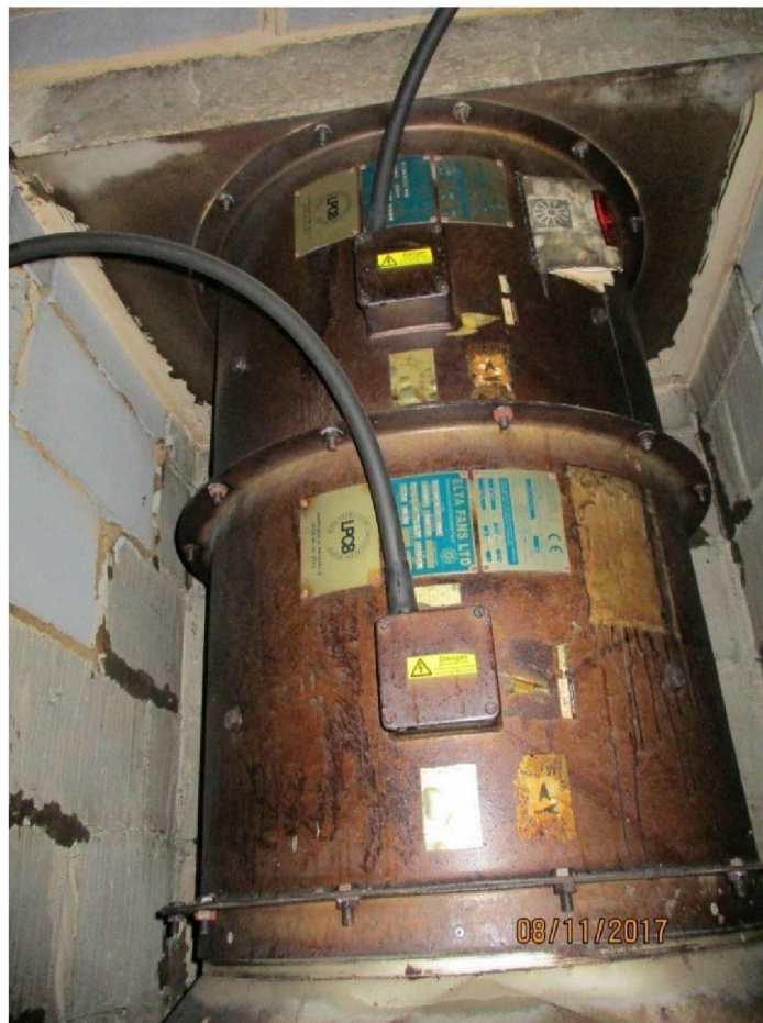
Figure J.12: Environmental / Smoke ventilation fans in the roof plant room
