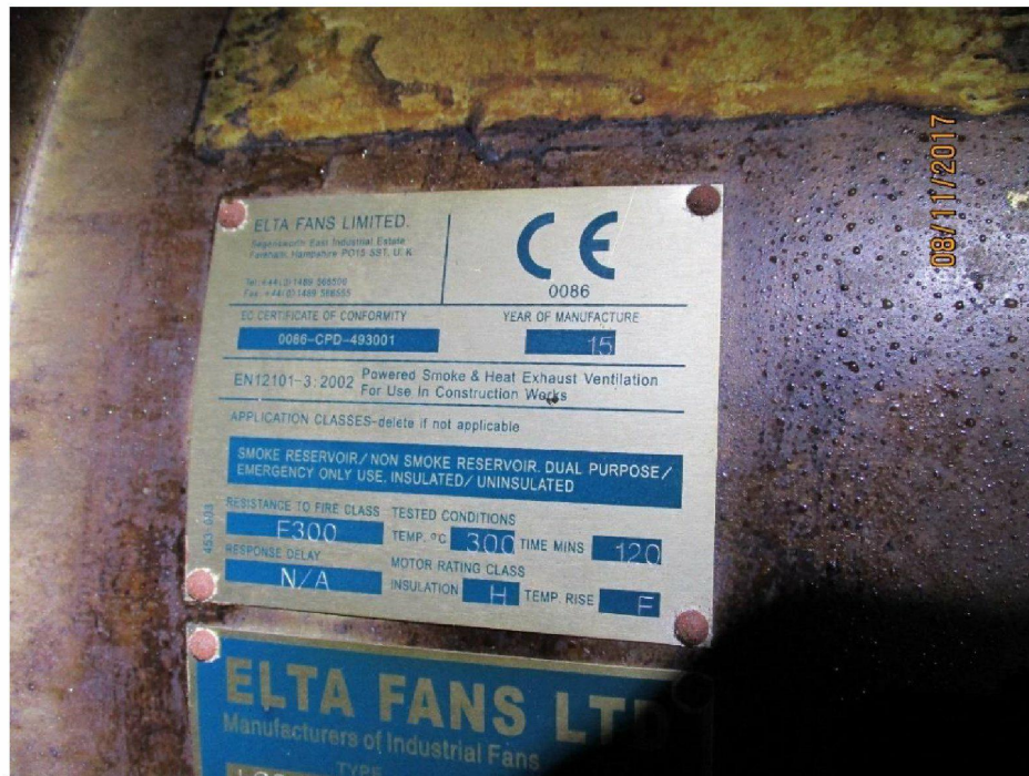
Figure J.14: Post fire inspection of fan information plates
