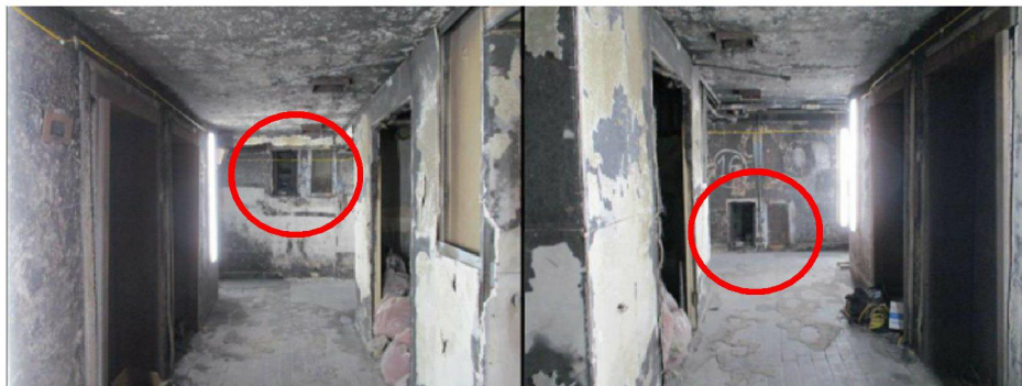
Figure J.10: Location of the AOVs in the Level 16 lobby. Left - North AOVs located at high level. Right – South AOVs located at low level.
