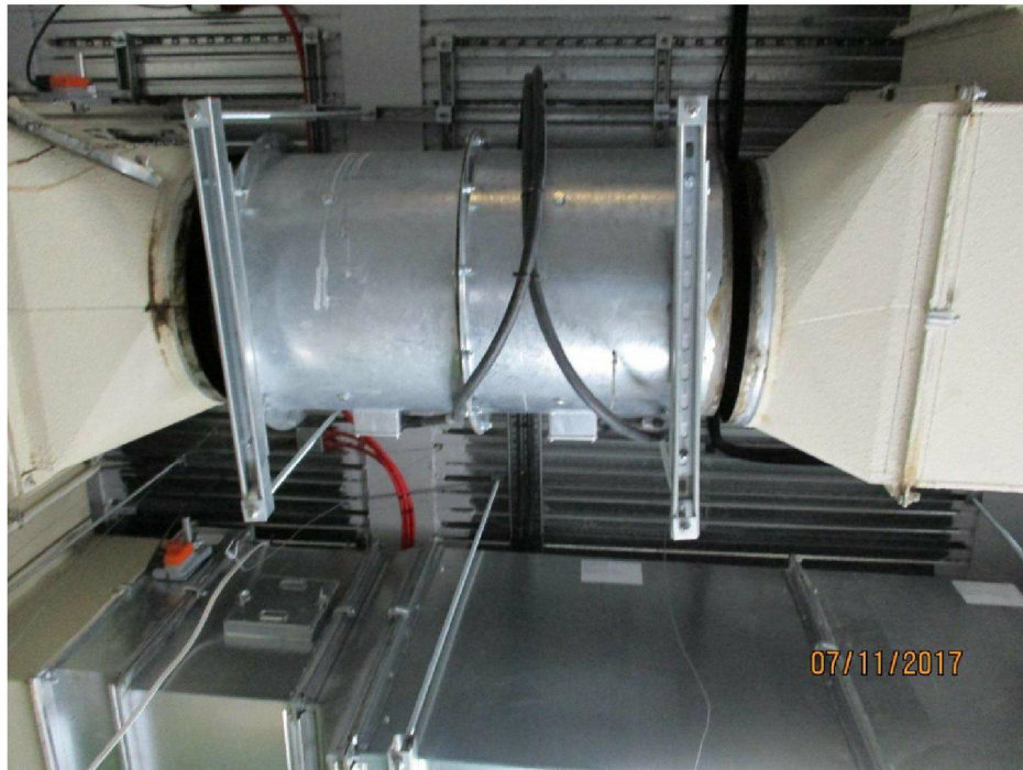
Figure J.13: Smoke exhaust fans at Level 2
