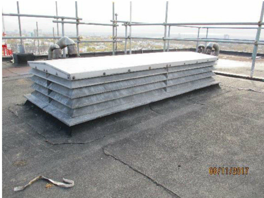
Figure J.9: Permanently open vent at Roof Level.
